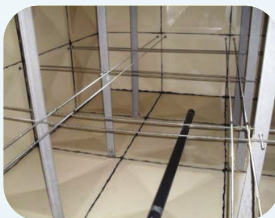
After showing replacement roof support structure
